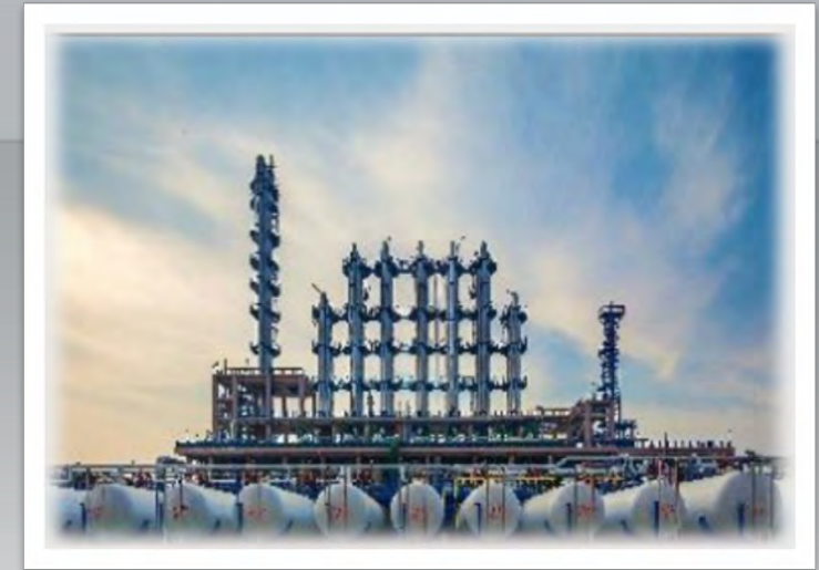
Xinhua Electronic Grade Polysilicon Production Plant
